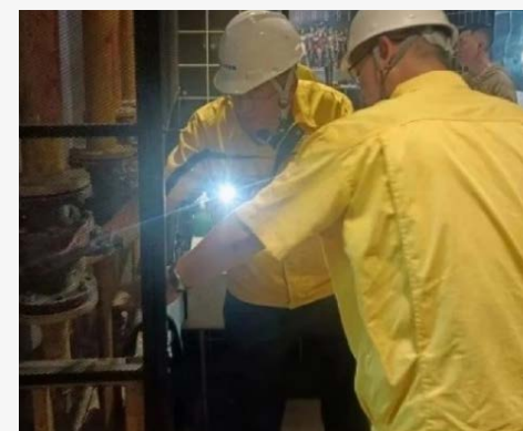
Potential safety hazard inspection by ENN Energy's personnel
