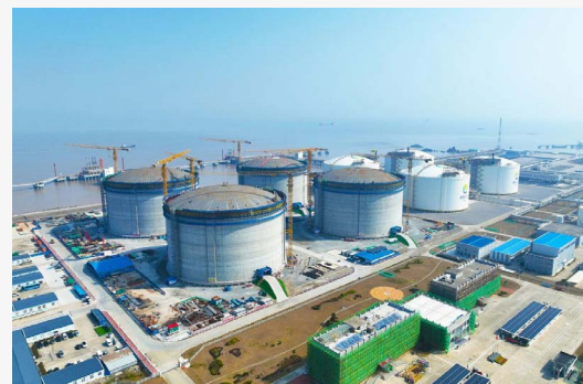
Bird's Eye View of Zhoushan Terminal Phase III Construction Site
